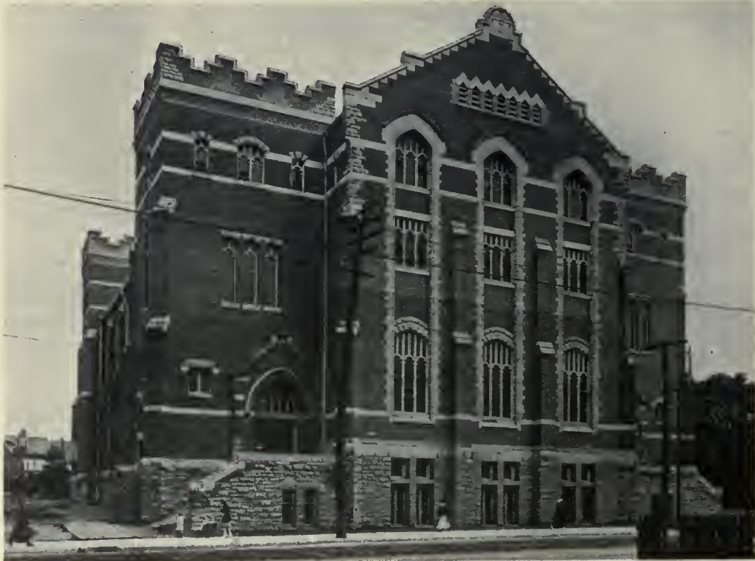
Fig. 1—Dale Presbyterian Church, Queen St. and Bellwoods Ave., Toronto.
